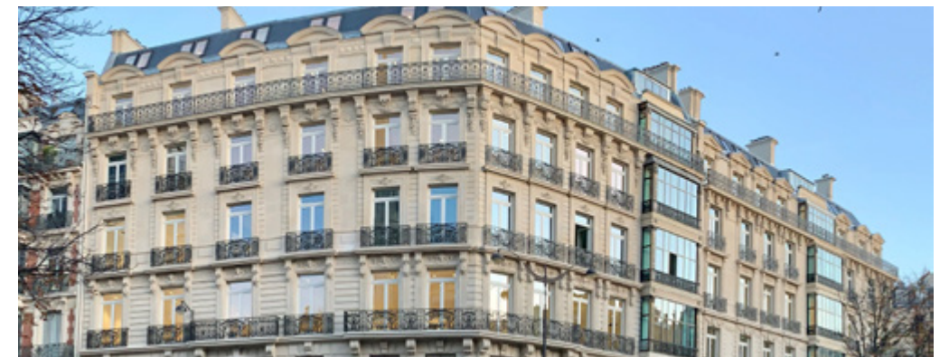
→ George V , Paris (75) - Brunet Gratio Architectes, JTPM Architecture
