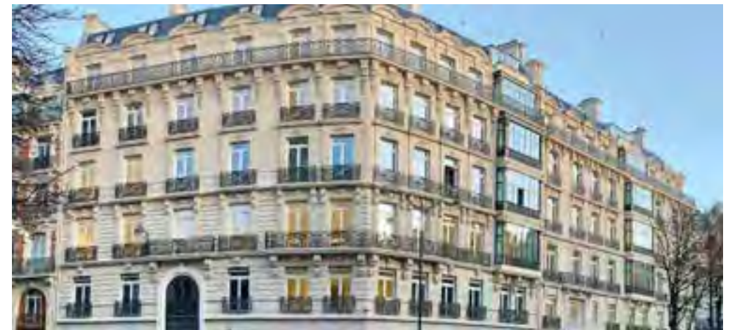
→ George V , Paris (75) - Brunet Gratio Architectes, JTPM Architecture
